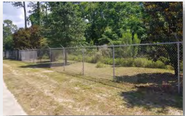
South Stormwater Pond
