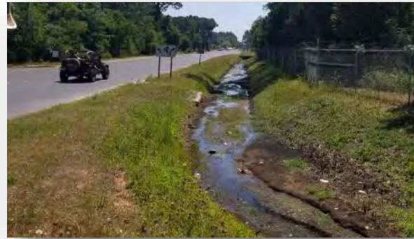
Culvert along Lovejoy Rd
