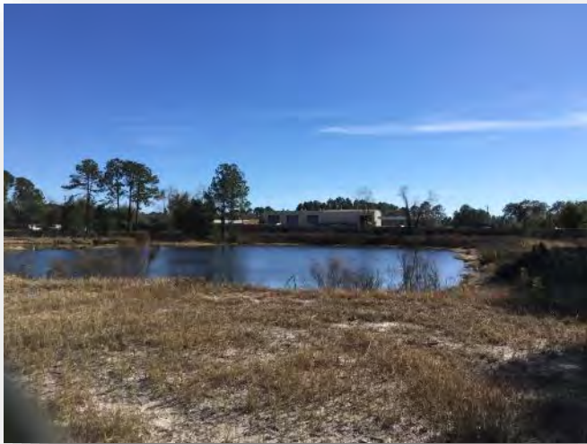
North Stormwater Retention Area
