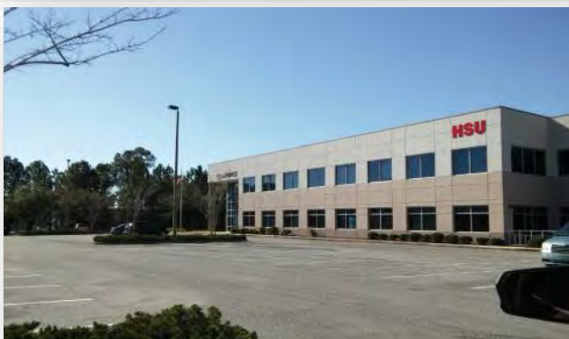
HSU Building along Ready Avenue
