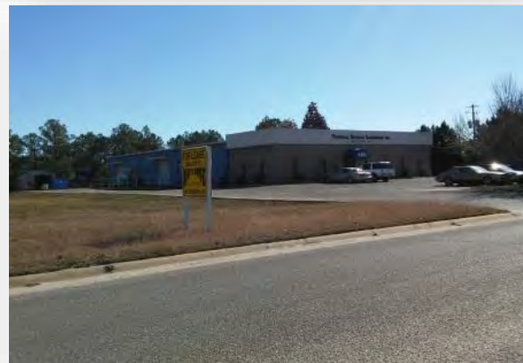
Existing Building along Ready Avenue
