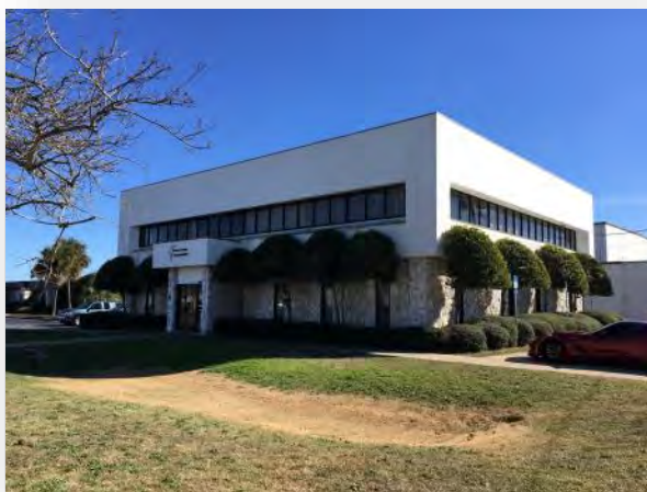
Vacant Office Building—Anchors St
