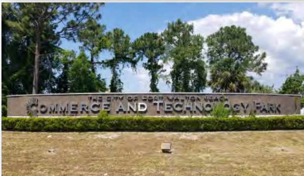
Existing Gateway Signage
