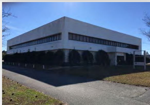
Vacant Building along Anchors Street
